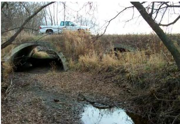
**Figure 2.59** The culvert on the left is Minimally Acceptable with sediment accumulation within the culvert. The culvert on the right is totally unacceptable with 2/3 of its flow capacity reduced by sediment and debris. This project was rated as UNACCEPTABLE because of the reduced flow capacity of the culverts. (MN)
