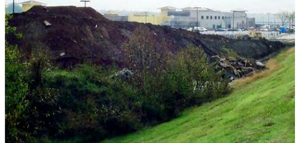
**Figure 2.10** UNACCEPTABLE, unapproved encroachment. Material stockpiled against the levee. (OK)
