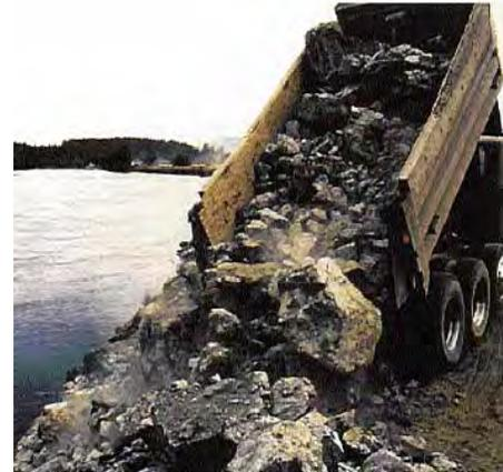
**Figure D.10** Placement of Riprap. Careful use of an excavator may allow for more accurate placement than is shown above.
