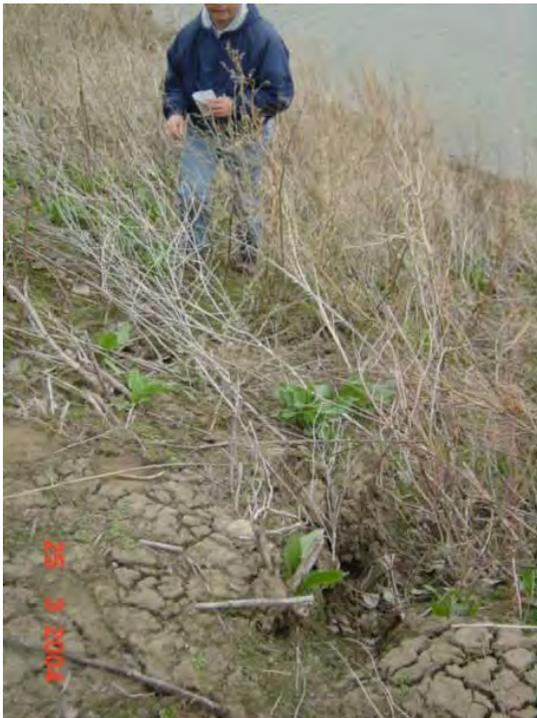
**Figure 2.34** *UNACCEPTABLE* cracking with landside pooling, Whitehead Levee Project, (IA)
