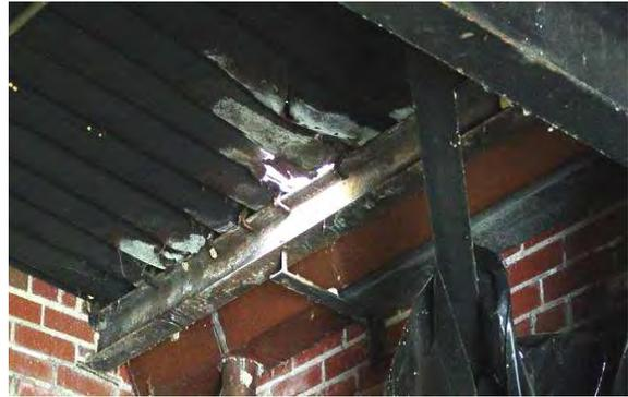
**Figure 2.67** Hole in roof of pumping station. (IL)
