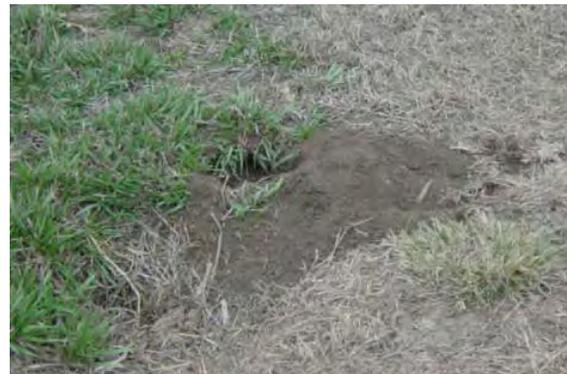
**Figure 2.20** Animal burrow in a levee. (IA)
