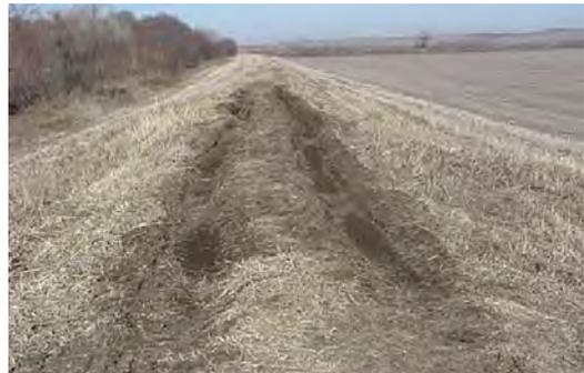
**Figure 2.37** *UNACCEPTABLE* ruts in levee crown require fill. (MO)
