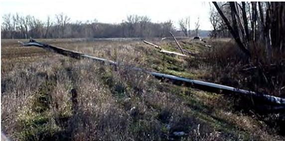
**Figure 2.9** UNACCEPTABLE encroachments on earthen levee. Fallen woody debris requires removal. (KS)
