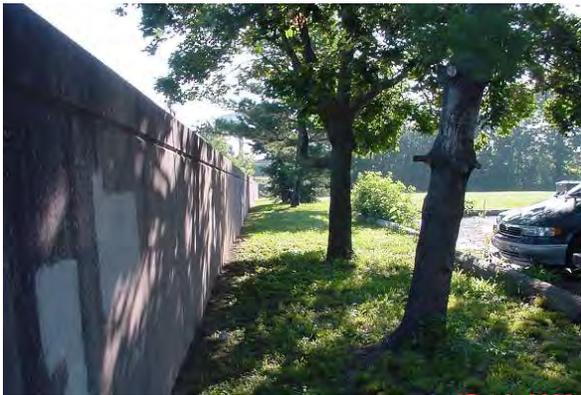
**Figure 2.51 UNACCEPTABLE.** *Trees growing too close to floodwall. (KY)*
