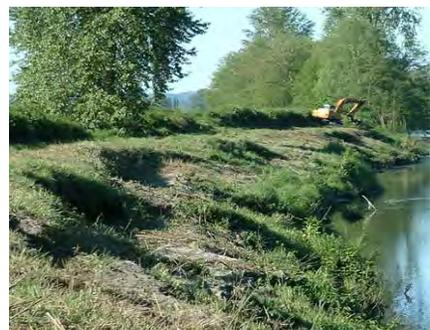
**Figure 2.3** *Slope failure on bank protection project. (WA)*
