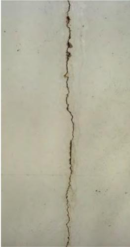
**Figure 2.43** *MINIMALLY ACCEPTABLE* 1/8<sup>th</sup> inch crack extends through concrete floodwall and needs to be sealed to prevent further damage. (MN)
