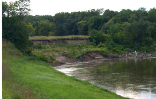
**Figure 2.16 UNACCEPTABLE.** Slope failure and erosion on a channel improvement project. (MN)
