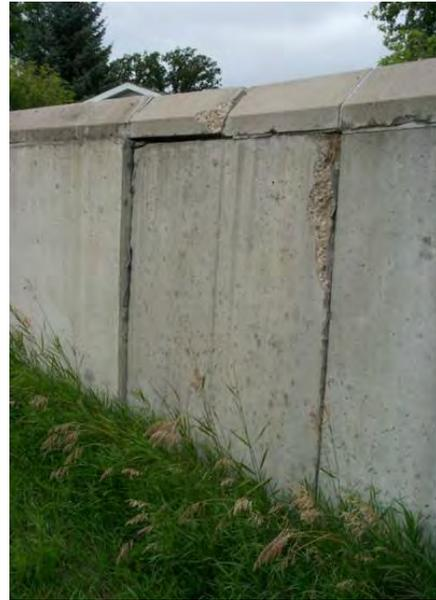
**Figure 2.49** *UNACCEPTABLE* monolith movement in floodwall. The monolith shown in the photo has tilted about 6 inches riverward as well a vertically. Note the movement when compared to the adjoining monolith and the top cap. As the monolith moved considerable spalling has occurred along the joint. This project is monitored very closely during flood events. (ND)
