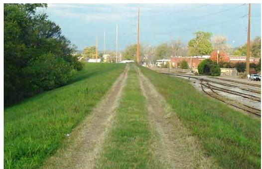
**Figure 2.39** *UNACCEPTABLE* rutting in levee. (OK)
