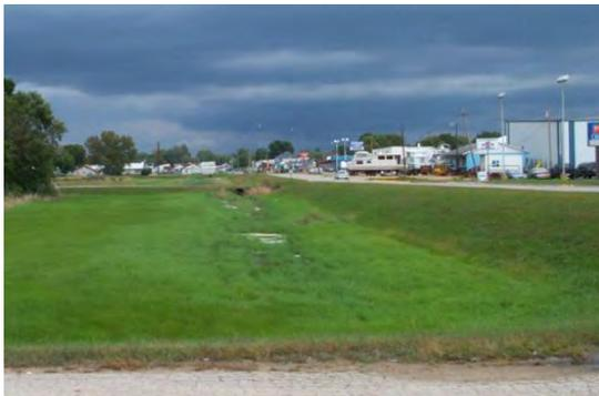
**Figure 2.54** *ACCEPTABLE interior drainage channel. (IA)*
