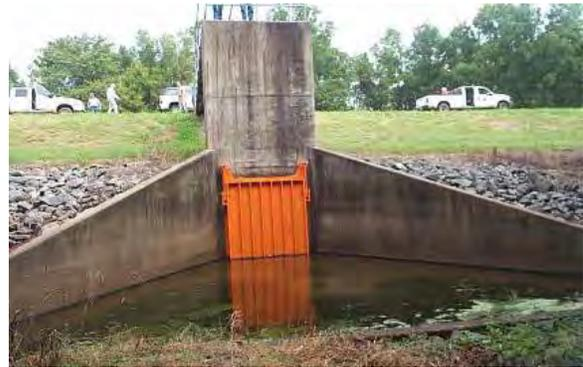
**Figure 2.63** ACCEPTABLE culvert gate. (LA)
