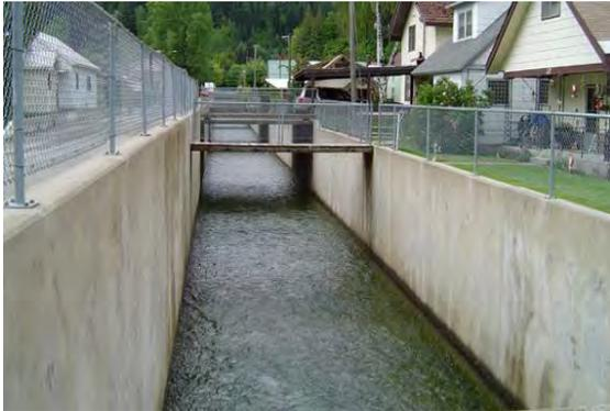
**Figure 2.72** ACCEPTABLE concrete lined flood control channel. (ID)
