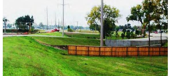
**Figure 2.12** UNACCEPTABLE, unapproved encroachment on levee easement (fencing). (OK)
