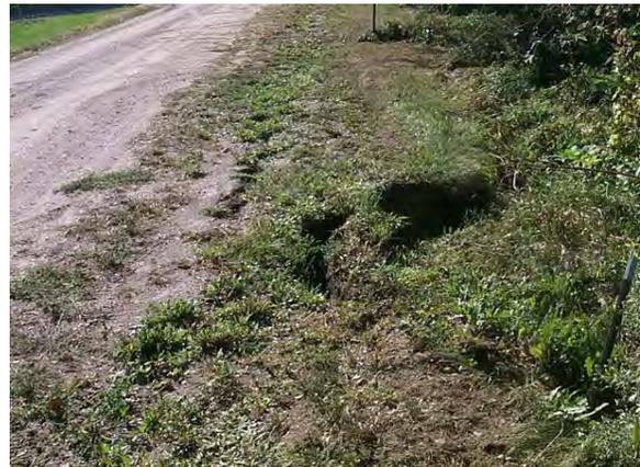
**Figure 2.35** *UNACCEPTABLE* embankment cracking and slope failure. This photo shows what started out as cracking along the crest of the embankment and quickly developed into a slope failure. All cracking located on a levee or riverbank must be closely monitored. (MN)
