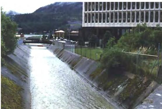
**Figure 2.74** ACCEPTABLE concrete lined channel. (AK)
