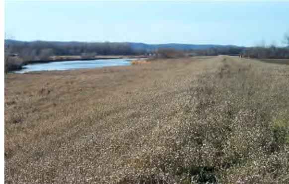
**Figure 2.30 UNACCEPTABLE** levee with knee-high grass, making visual inspection nearly impossible. (MN)
