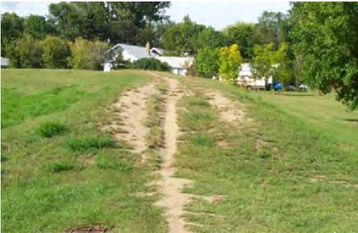
**Figure 2.36** *MINIMALLY ACCEPTABLE* levee rutting caused by pedestrian and bicycle traffic. (ND)
