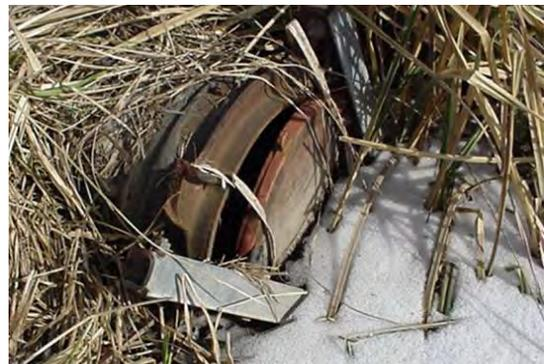
**Figure 2.66** UNACCEPTABLE flap gate in earthen levee. (Broken hinge and vegetation growth.) (MO)
