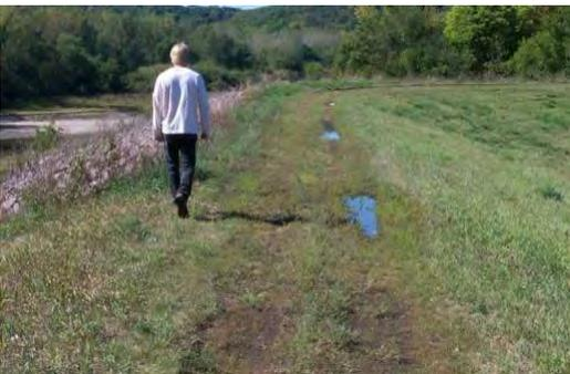
**Figure 2.38** *MINIMALLY ACCEPTABLE* ponded water along a levee crest. (MN)
