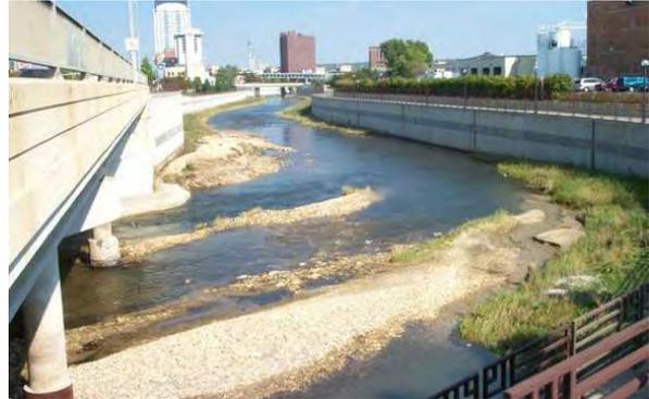
**Figure 2.71** *MINIMALLY ACCEPTABLE* shoaling within a concrete lined channel. (MN)
