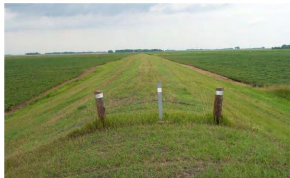
**Figure 2.5** *MINIMALLY ACCEPTABLE*. Field encroaches on levee easement. The landowner has tilled the soil right to toe of the levee, and was requested to stay back at least 10 feet. (ND)
