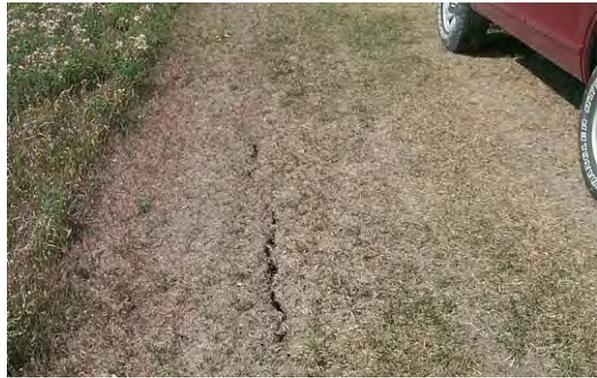
**Figure 2.33** *ACCEPTABLE* cracking in clay levee with shrinkage cracking caused by dry conditions. (MN)
