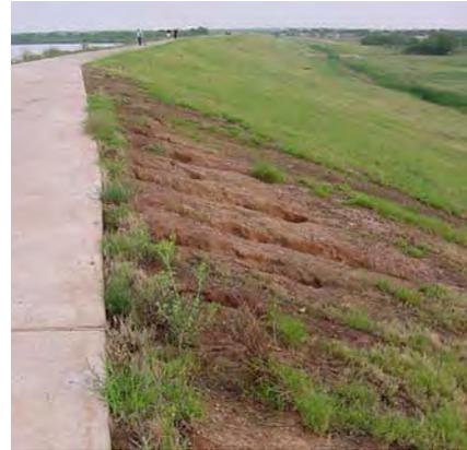
**Figure 2.1** *UNACCEPTABLE erosion of levee slope. (TX)*
