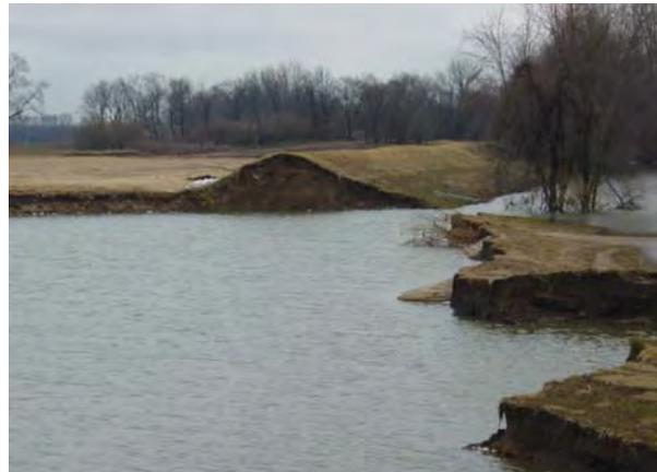
Figure 6.2 and 6.3, Levee breaches along the Wabash River
