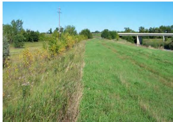
**Figure 2.32 UNACCEPTABLE** long grasses and trees on levee side slopes. (ND)
