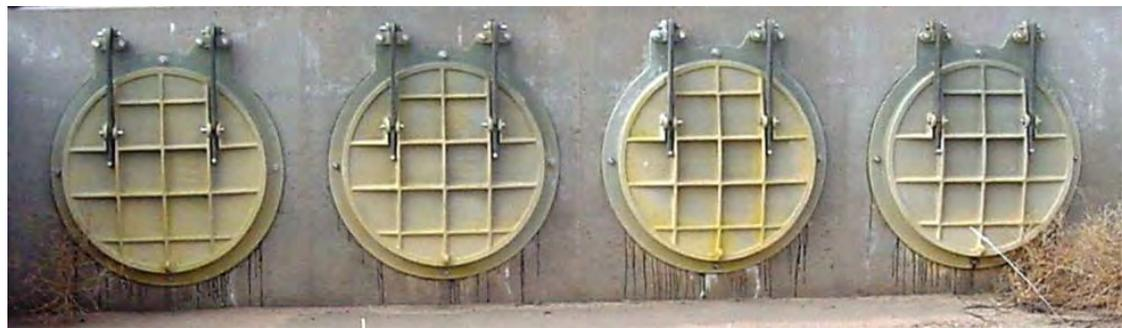
**Figure 2.64** ACCEPTABLE flap gates in earthen levee. (KS)
