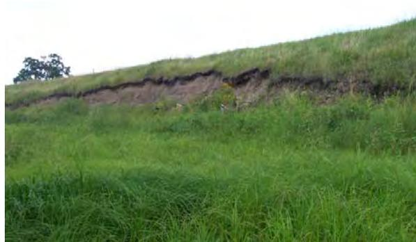
**Figure 2.17 UNACCEPTABLE** earthen embankment failure. (MN)
